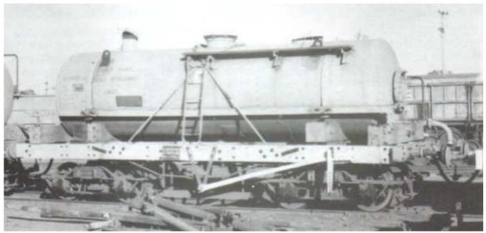
Queensland railways style fabricated bogies, all the bolt detail, interesting and unique.
